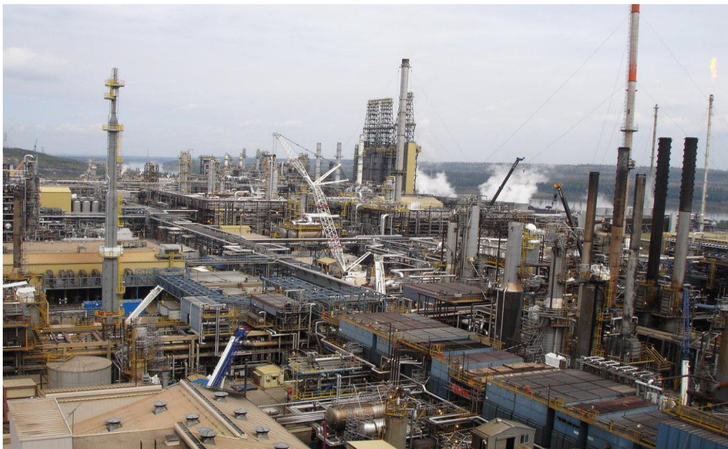
Figure 1.1 Oil and Gas Construction Project in Alberta, Canada Source: http://www.albertaenergychallenge.com/#!__main/page-2
