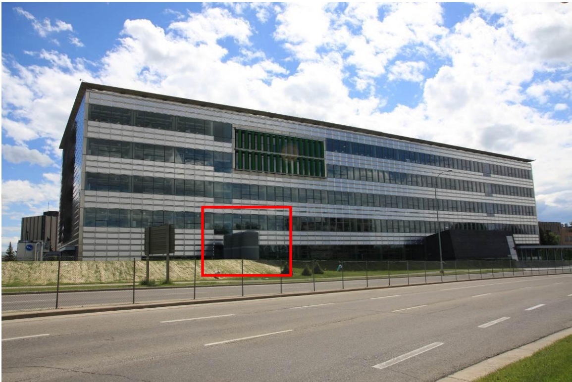
Figure 3.1 North Façade of the EEEL Building (the Earth Tube Intakes are Highlighted)
