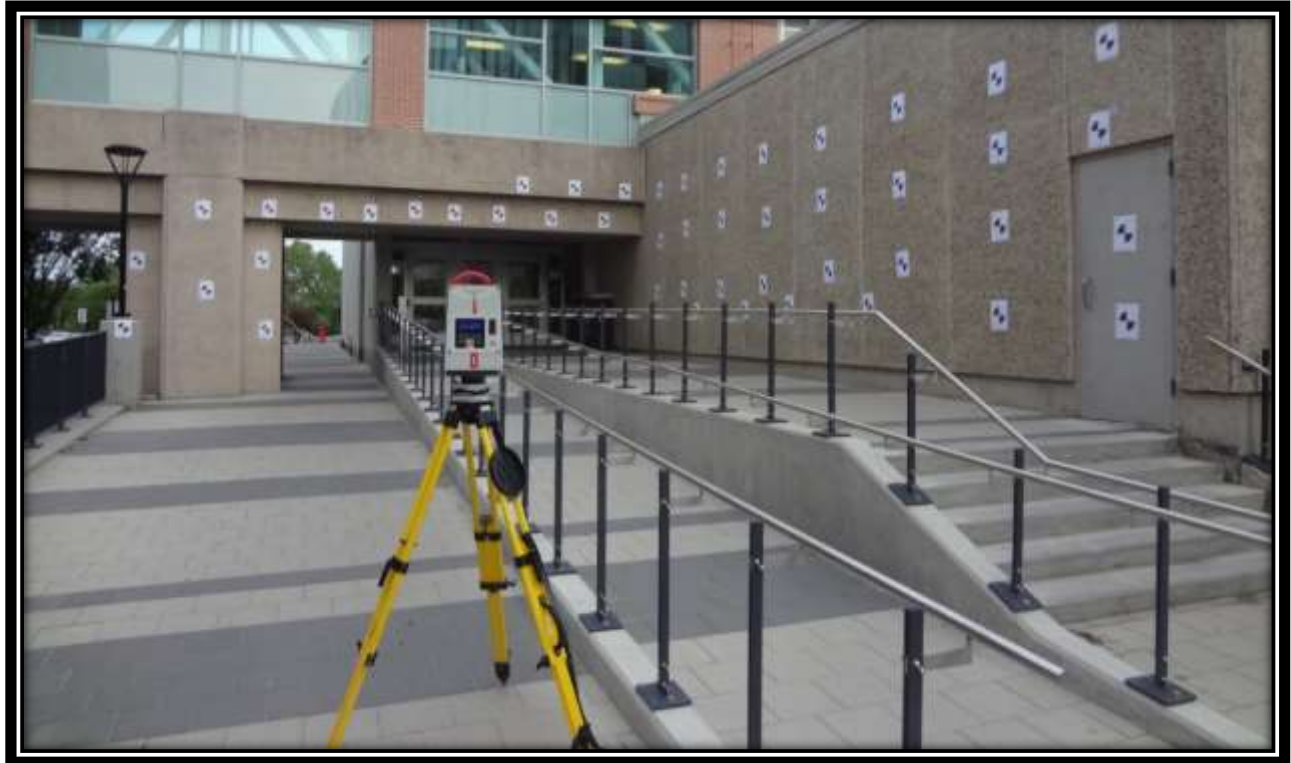
Figure 4-1: Image of the Northwest quadrant of the experiment site showing Leica black-and-white six-inch targets placed on walls at the University of Calgary (facing South)
