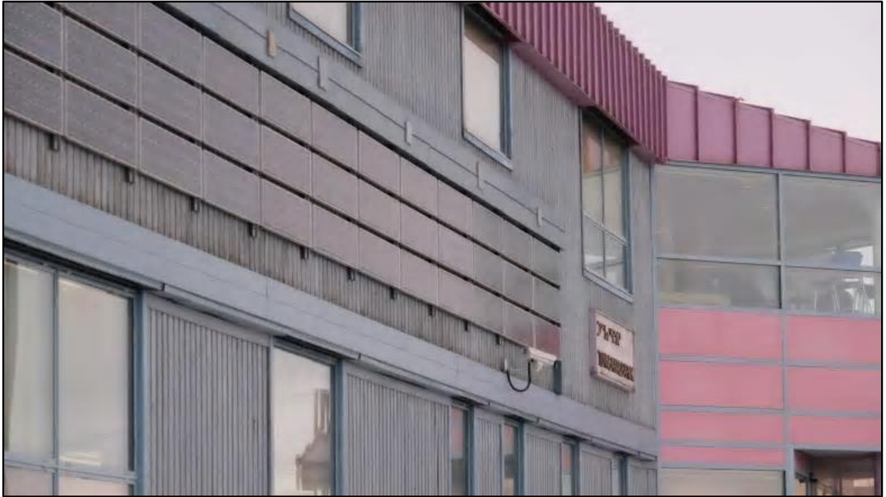
Figure 7: Solar PV Array vertically oriented on Arctic College in Iqaluit, Nunavut
