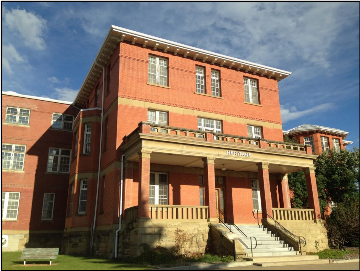
Figure 3.6. Photograph of the front of the Heritage (Main) Building at the Provincial Mental Hospital, Ponoka (now The Centennial Centre for Mental Health and Brain Injury). The photograph was taken by the author (B.M. Collins) in August of 2014.
