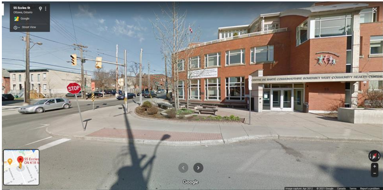
Somerset West Community Health Centre April 2012(Before SCS)
