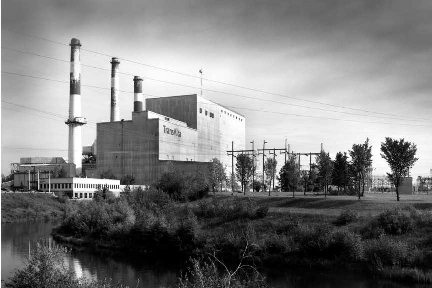
WABAMUN POWER PLANT (TRANSALTA).
