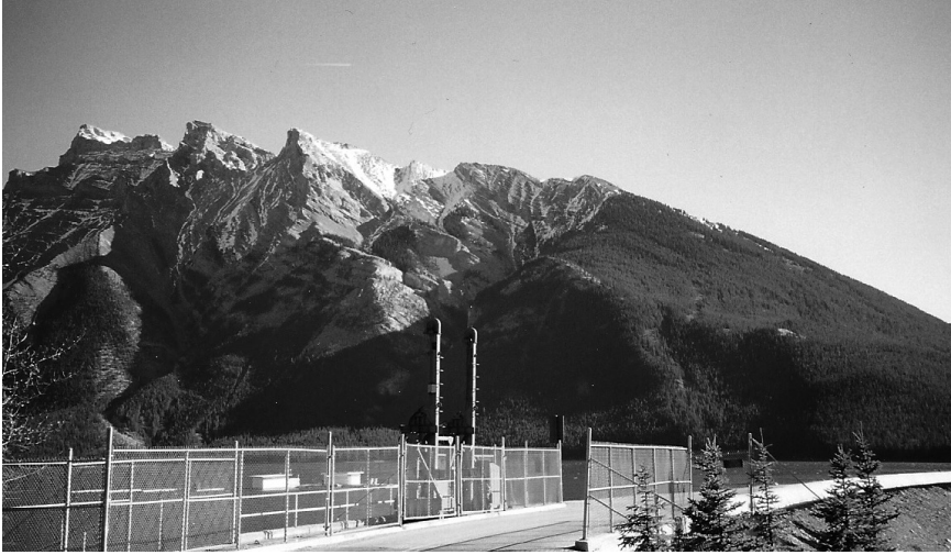
1941 DAM AT LAKE MINNEWANKA (AUTHOR PHOTO).
