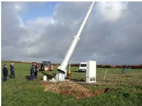
Figure 24: Monopole Tower (youtube, 2010) with hydraulic system for raising and lowering
