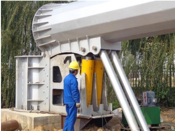
Figure 25: Hydraulic support for the pole of Wind turbine (Hummer)
