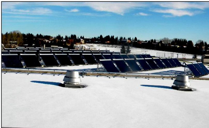
Figure 3.3: Spacing and Orientation of SLC ETC Panels. Photographed by Athaudage Dona, (2012)
