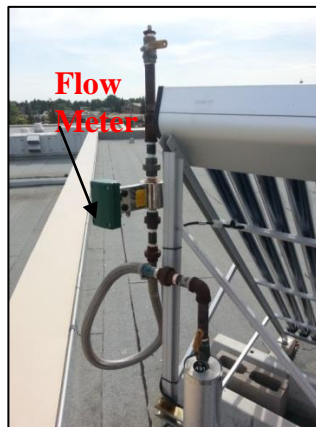
Figure 3.10: Flow Meter Vertical Installation Position from October 2012 to May 2013.
