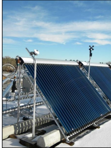
Figure 3.2: Heat Pipe Evacuated Tube Collector: Photographed by Athaudage Dona, (2012)
