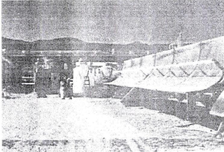
**Figure 1.2 Parabolic Trough Solar Concentrating Collector (Goswami et al., 2000)**
