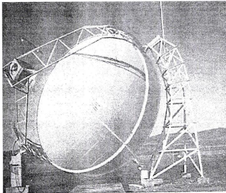
**Figure 1.3 Compound Curvature Concentrating Solar Collector (Goswami et al., 2000)**
