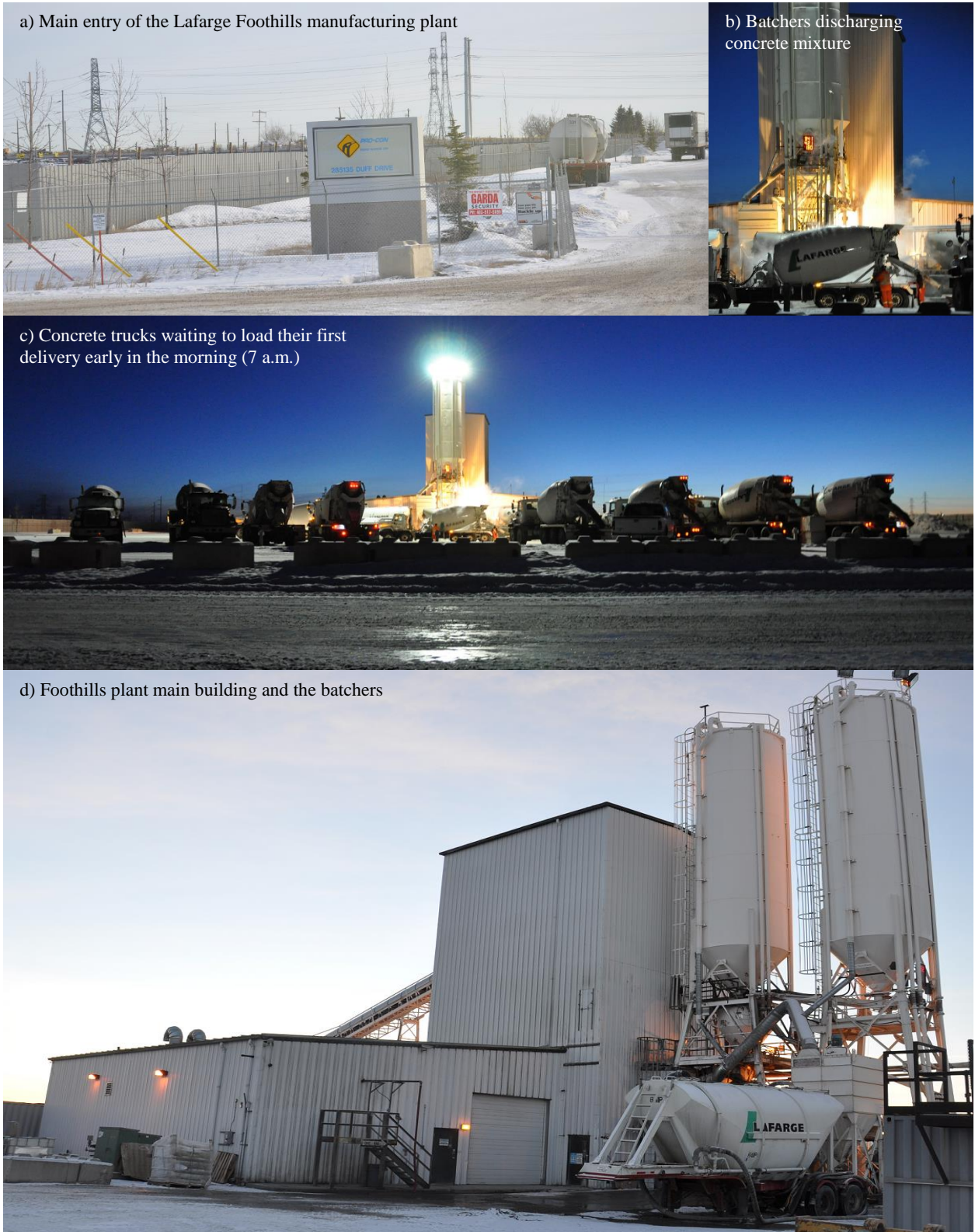
Figure 5-2 Foothills ready-mix concrete manufacturing plant
