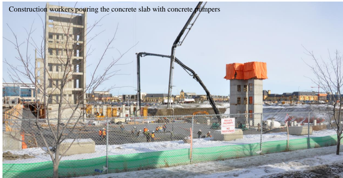
Figure 5-3 Quarry Park construction site
