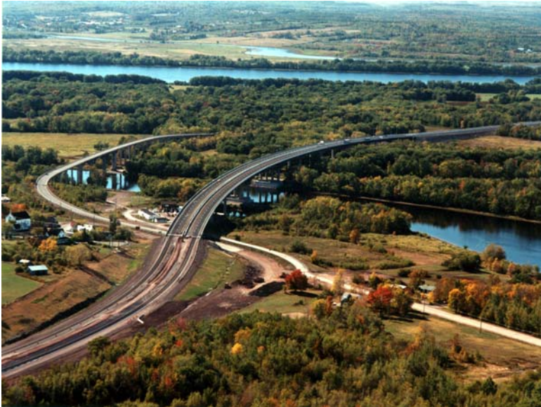
Jemseg River Bridge
