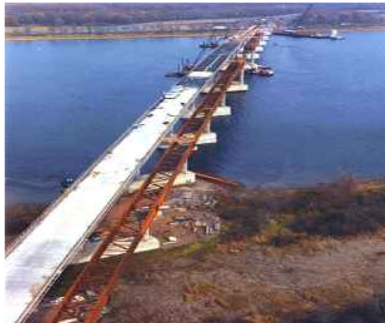
Saint John River Bridge
