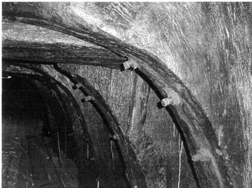
Figure 13. Oak beams at upper gundeck inside the Vasa, showing some corroding iron bolts. The white lines are from surplus PEG4000 from the surface treatment.
